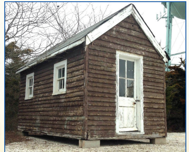
During the restoration process, shingle siding was removed to expose original clapboard.
