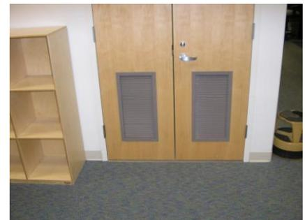
**Louvers were installed on the doors to the technology closet to increase airflow into the area**
